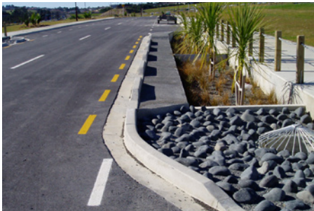
Rain Garden at Albany Park and Ride station showing the slotting curb allowing storm water inflow and outflow structure
