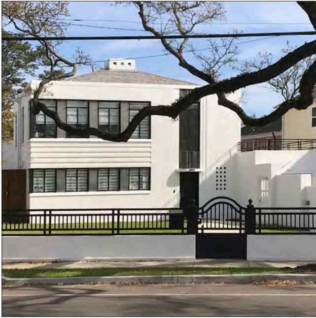
The horizontality of the modern style is visible in the ribbon windows as well as the decorative banding that wraps the corner of this residence.
