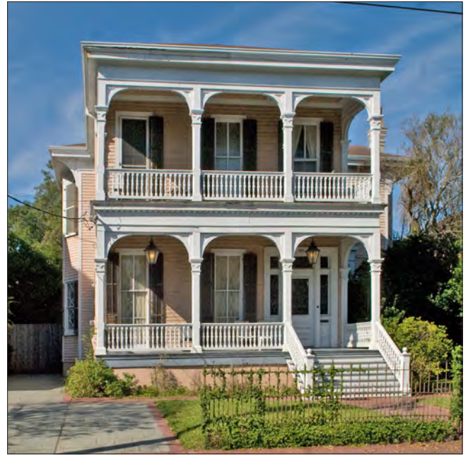
The posts supporting the double gallery have arched brackets and a deep horizontal overhang, typical of the Italianate style.
