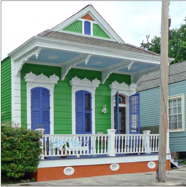
This bracketed shotgun house has Italianate brackets supporting the deep front overhang above.
