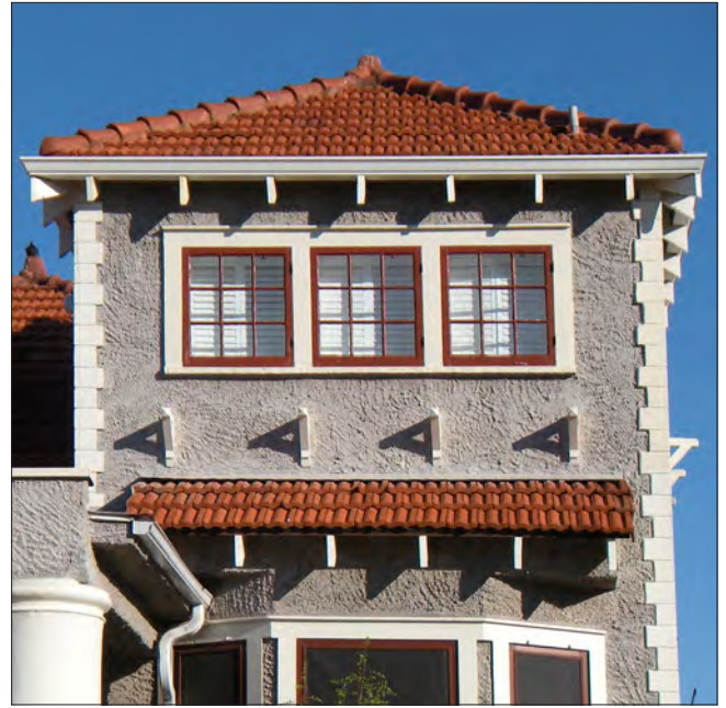
This corner tower feature has a pyramidal hipped roof covered with red terra cotta tiles. The textured stucco walls are framed by smooth "quoins".
