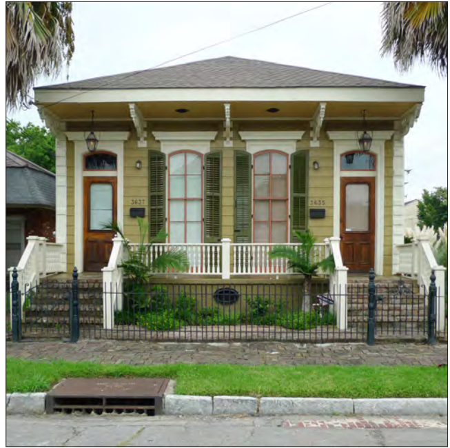
The form of this residence is typical of a double Shotgun with a central pair of windows flanked by entrance doors.
