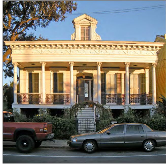
This raised Center Hall Cottage is spanned by a deep front porch.
