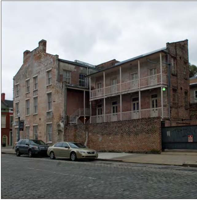
The main block of this Townhouse features a side gable roof. Townhouses typically include multi-level service wings accessed by exterior galleries.
