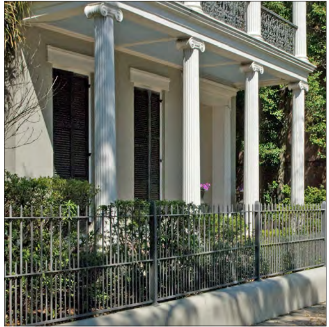
This double gallery is supported by fluted Ionic columns which are more delicate in appearance than the square posts typically associated with Greek Revival buildings.
