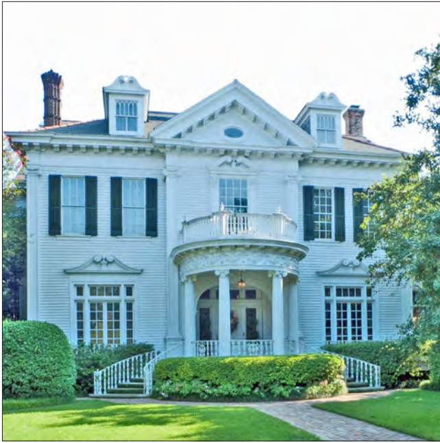
Neoclassical buildings often feature classically inspired details such as fluted porch columns, ornate cornices and pediments.
