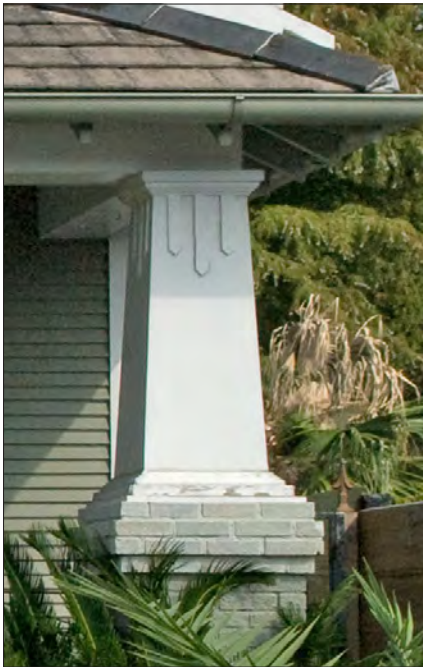
This high-style Arts and Crafts home features exposed rafter tails and fascia boards, various wood siding finishes and deep porches and overhangs.
