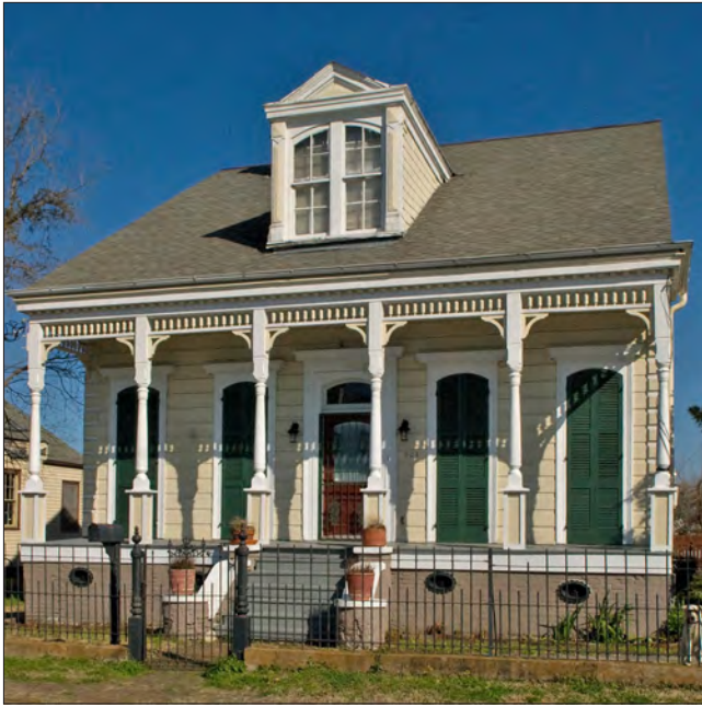
The side gable roof form, central door flanked by windows and deep front porch are typical features of a Center Hall Cottage.
