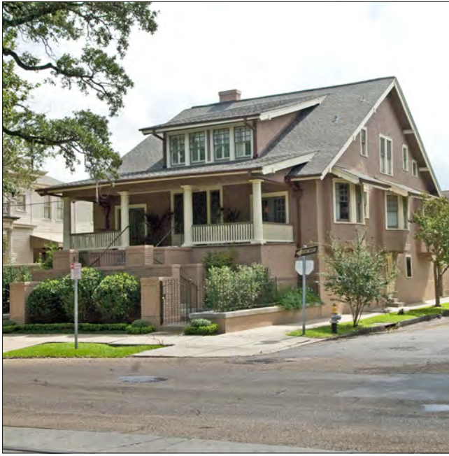
The prominent shed roof dormer with multiple windows, extended eaves, and deep front porch are typical of a Bungalow.
