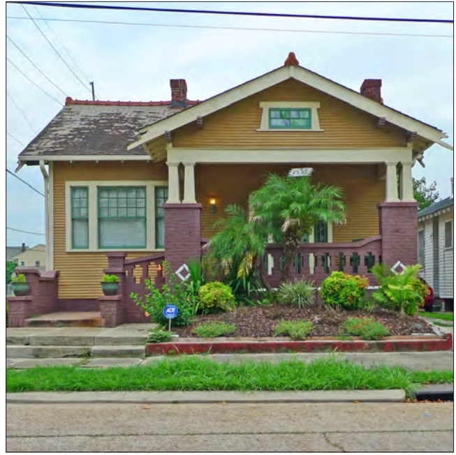
This Bungalow features intersecting roofs with overhanging eaves as well as a deep porch.
