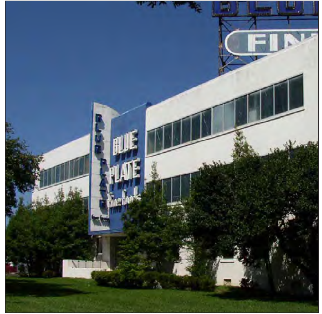
This plain concrete buildings feature continuous ribbon windows with chrome frames, which are interrupted by the central, decorative neon wall and blade signs.
