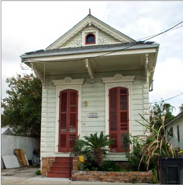
This narrow single Shotgun includes a paired, shuttered, door and window with a front gabled roof and a hipped projecting overhang.
