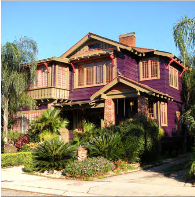
This high-style Arts and Crafts home features exposed rafter tails and fascia boards, various wood siding finishes and deep porches and overhangs.
