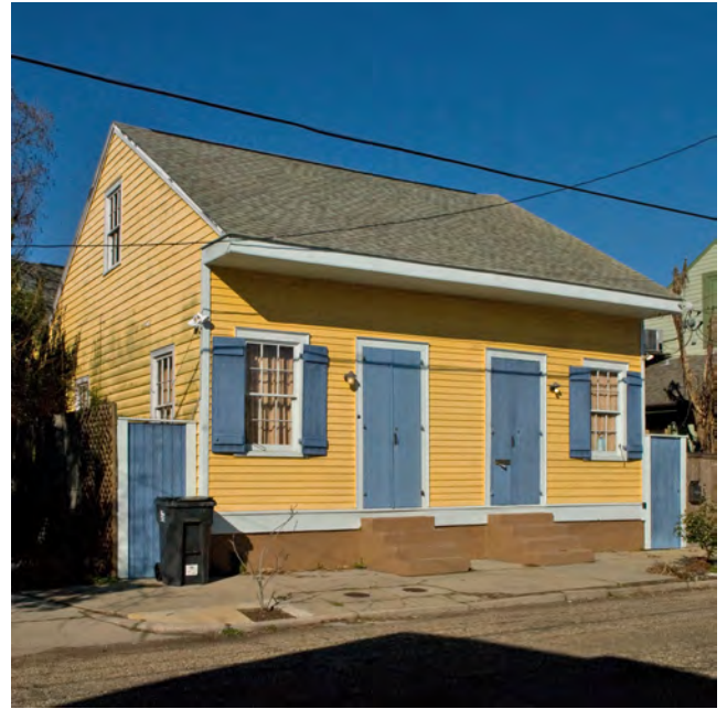
This weatherboard Creole Cottage has a steeply pitched side gable roof that extends over the front façade to provide rain protection over the windows and doors.
