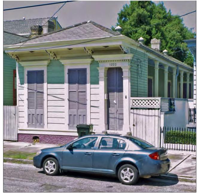
This Side Gallery Shotgun features a narrow covered side porch at the right that acts as an exterior corridor to connect the rooms.
