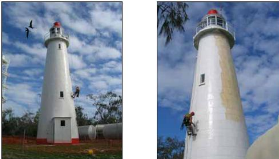
Figure 6. Lighthouse maintenance in 2007 (Images: Wayne Fox)
